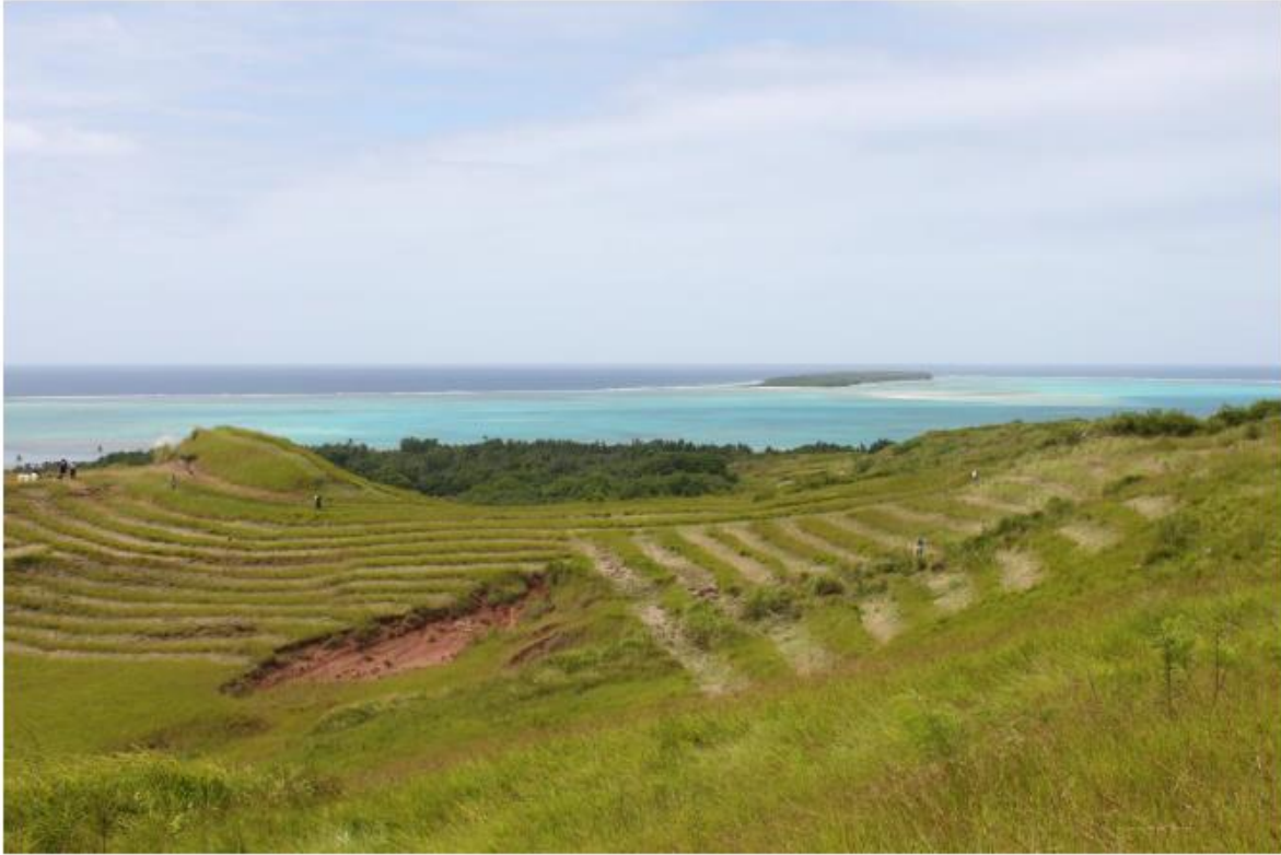
Site preparations in a High Priority Area.
